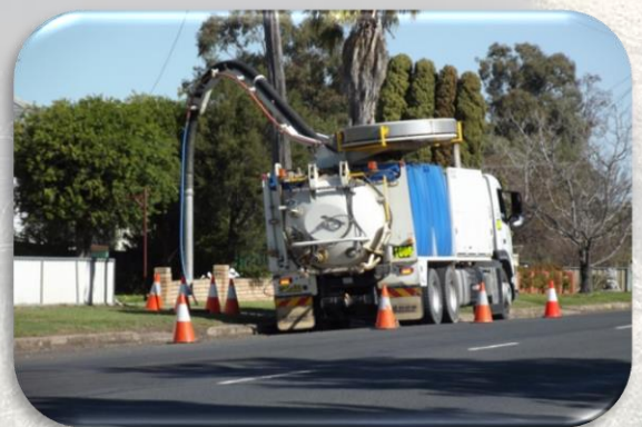
Sewer pipeline cleaning and CCTV inspection work
