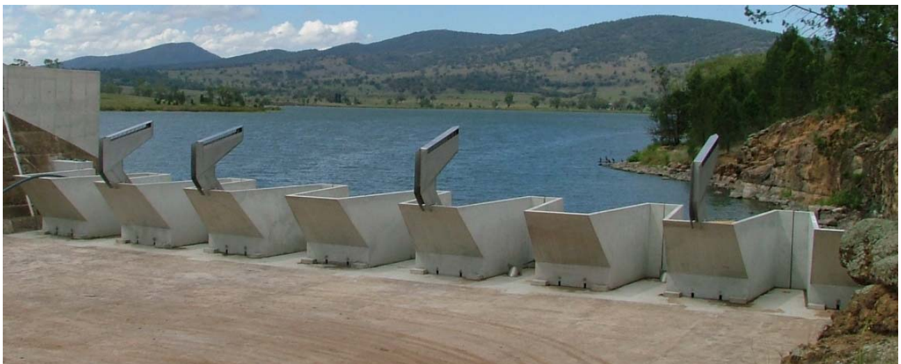
Fusegates on the spillway – Quipolly Dam Upgrade
