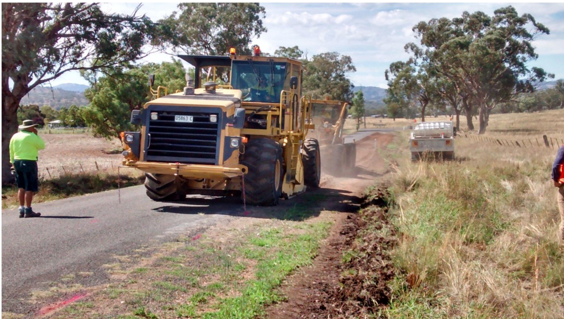
Heavy patching using a pavement stabilizer to mix cement with the gravel
