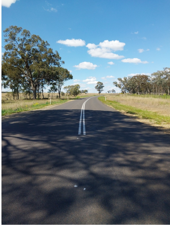
Figure 8: Looking East from Wandobah Rd intersection
