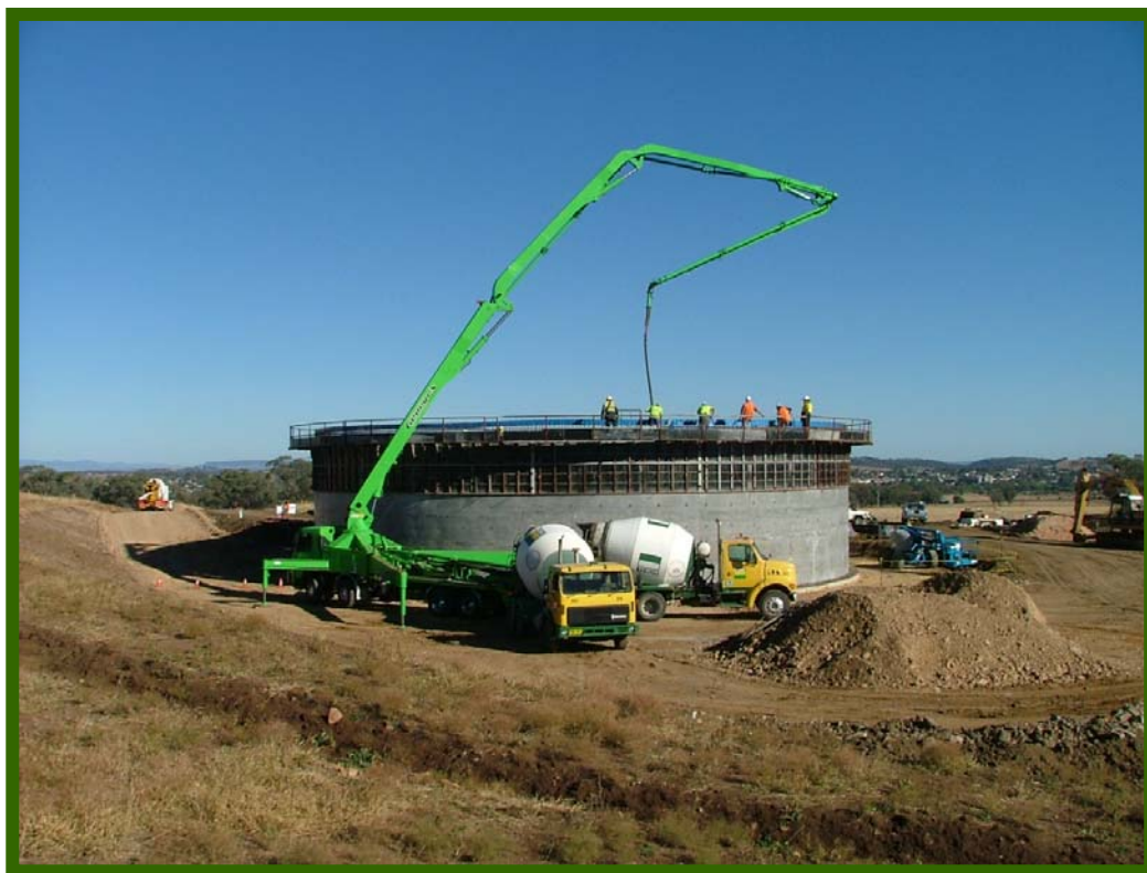
Construction of the new 5 Million Litre Reservoir East of Quirindi
