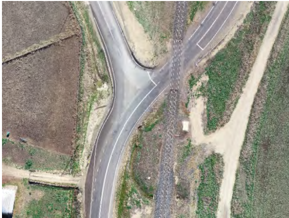
Plate 17 - Werris Creek Road level crossing aerial view
