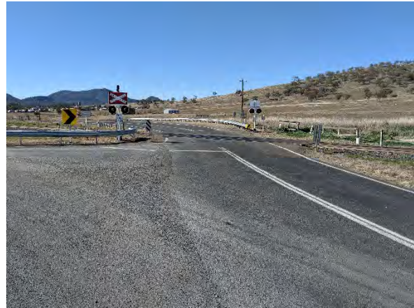
Plate 18 - Werris Creek Road level; crossing looking north-east
