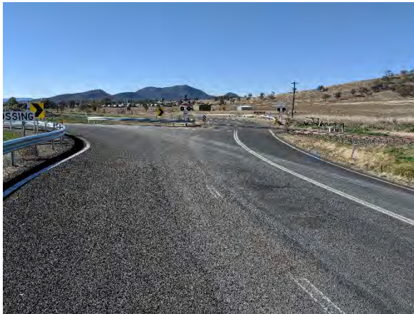
Plate 11 - Werris Creek Road looking north-east towards level crossing and intersection
