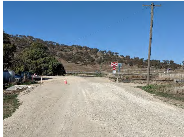
Plate 2 - Road narrowing on South Street at culvert
