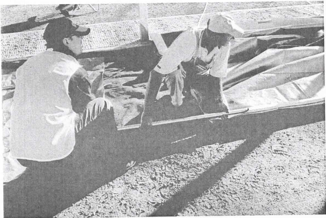
INSERTING TARP PIPES
